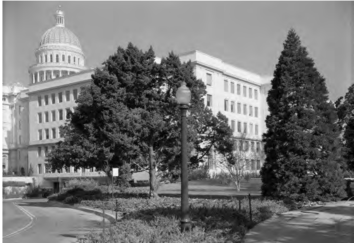
1952 CAPITOL ANNEX BUILDING Demolished Apse and Impacted Dome Views
