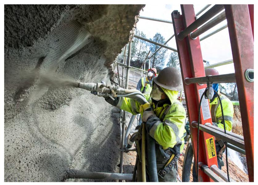
March 5, 2017 Specialized concrete is applied below the lip of the damaged Oroville Dam flood control spillway
