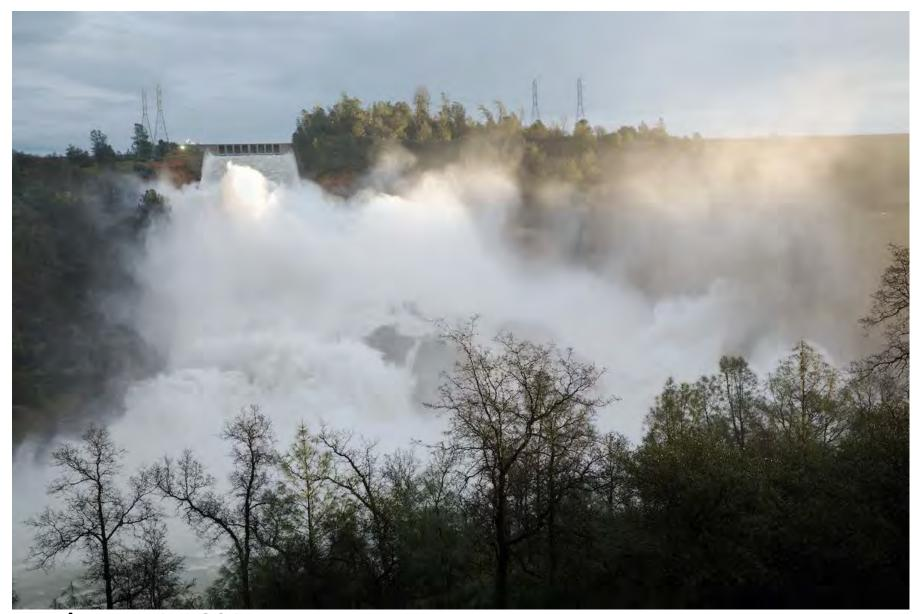
**February 15, 2017** 100,000 cubic feet per second (cfs) of water was released over the damaged spillway
