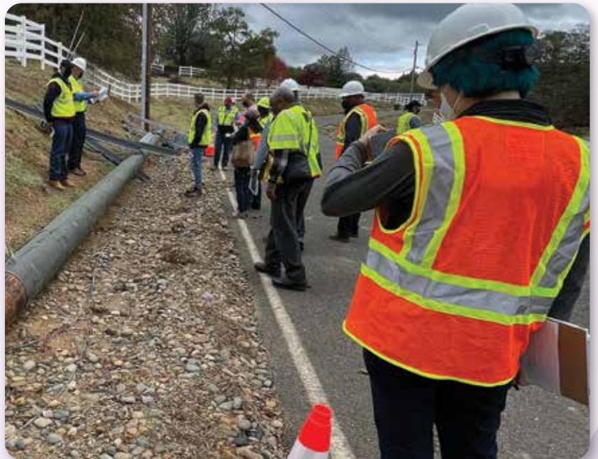
Reviewing a Covered Conductor Project in PG&E Territory.
