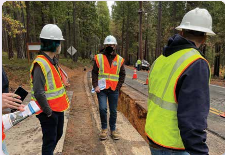
Inspecting an Undergrounding Project in PG&E Territory.
