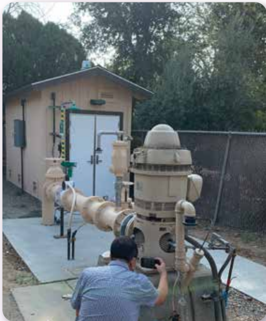
Inspecting Arden Cordova - Morse 8 Well.
