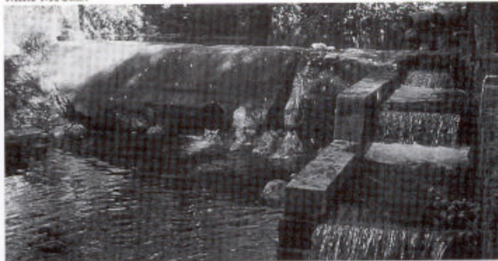
(Left) Monkey Creek Trout Haven Dam in California was removed earlier this year. The domestic water intake wall and ladder was left for support of the wall.
