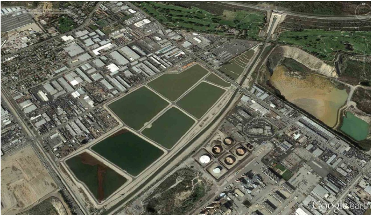
Hansen Spreading Grounds- Full (Aerial images courtesy of Google earth)
