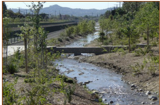
After construction — Completed 2007
