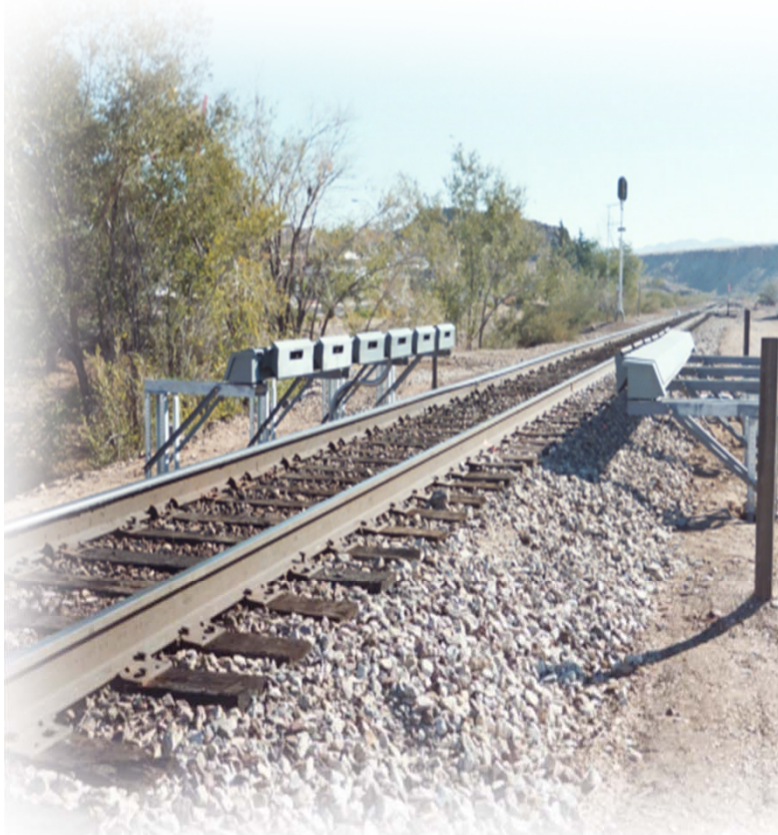
Acoustic Bearing Detector
