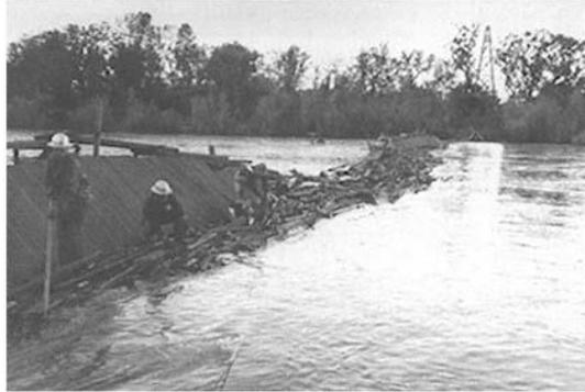
Best intentions weren't enough. High water in December 1941 washed out the fish trapping facility at Balls Ferry on the Sacramento River. Rebuilt in 1943, it was abandoned as unworkable within three years. This structure was part of the "Shasta Salvage Plan" to relocate salmon displaced by the construction of Shasta Dam.
