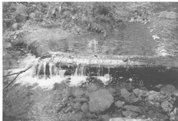
Small structure, big effect. Headwater stream restoration by artificial placement of stone or log deflectors adds oxygen to the water and provides protective rearing habitat for juvenile salmonids. Thousands of such structures are being built on California river tributaries.
