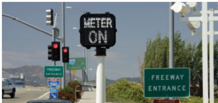
Caltrans programmed freeway onramp traffic lights to alternate so cars merge once onto the freeway, eliminating the additional merge within the onramp.
