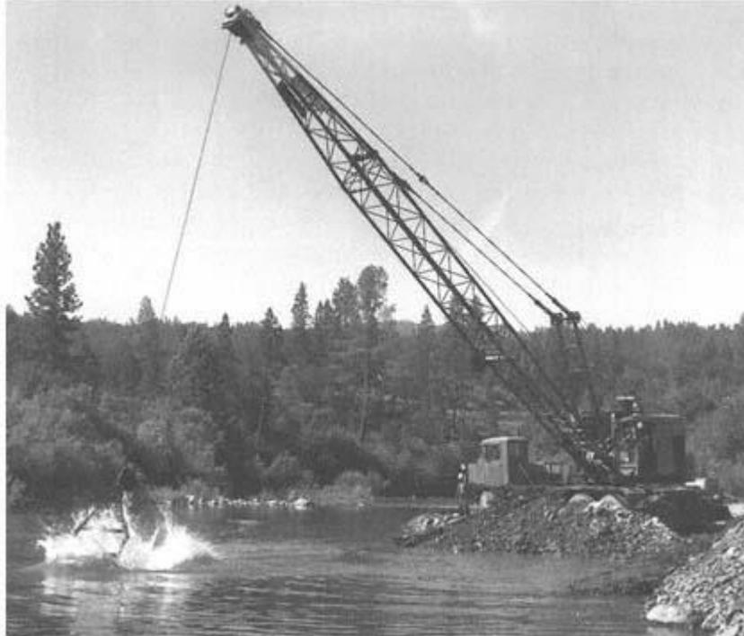
Cool water needed. Dredging, equipment removing gravel to create cold water pools for protection of salmon and steelhead on the Trinity River.
