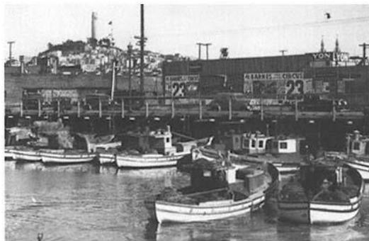
Monterey. The boats pictured in the 1930s at Fishermen's Wharf, San Francisco, were powered by one-cylinder gasoline engines. The Monterey replaced the sail-powered felucca in the California commercial salmon fishery.
