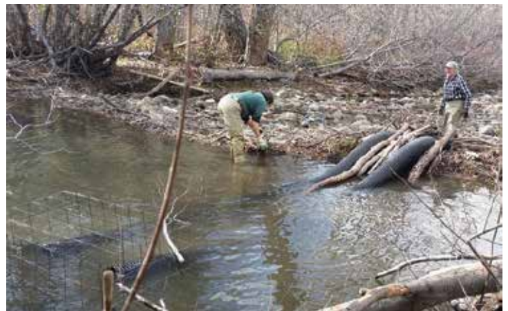
Sherry and Ted Guzzi of the Sierra Wildlife Coalition install a flow control device on Taylor Creek in South Lake Tahoe. (Photo: Sheri Harstein)
