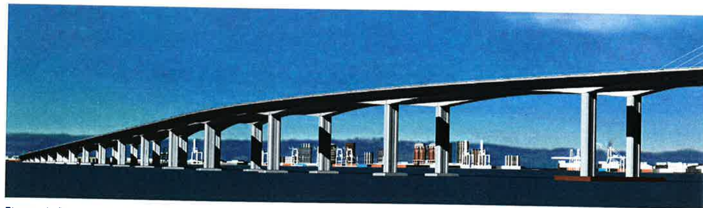
Figure 6. Panoramic View of Skyway with Haunched Concrete Girder
