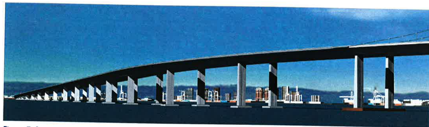
Figure 7. Panoramic View of Skyway with Uniform Depth Steel Girder
