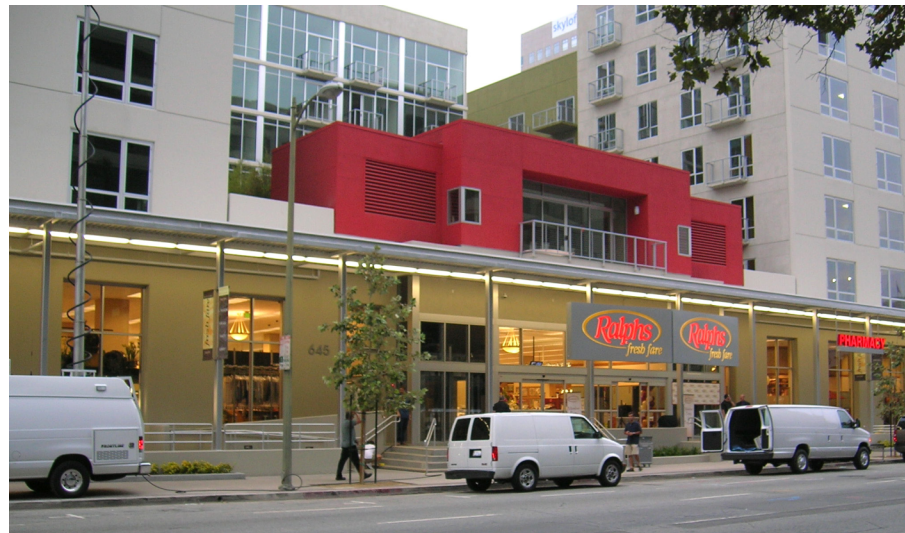
The Market Lofts: Los Angeles, California. LA's first supermarket in 50 years. Developed by CIM
